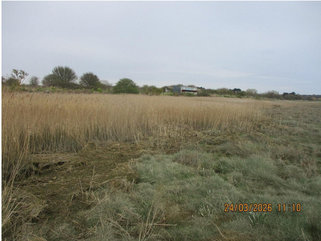
Photograph A1.15 Phragmites reed bed at the landward margin of the saltmarsh fronting the Pegwell Bay Country Park rock revetment, south of the bird hide
